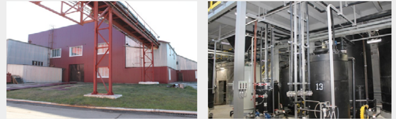
Figure 29. JSC Dalur's Pilot Commercial Production Unit (Central Section of Dalmatovskoye Deposit)
